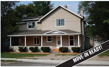
308 MAPLE • EAST JORDAN This 4BR home has been newly remodeled, has new flooring throughout and has been freshly painted. MLS 438295. Ask for Holly Nierman. $74,900
